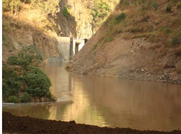
Omo River being diverted through one of the three diversion tunnels
